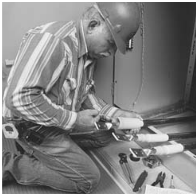
3M™ Cold Shrink QT-II Indoor Termination
